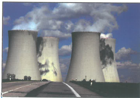
Power Plant - Cooling Towers
